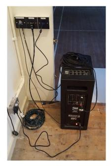
The left hand speaker, looking from the stage, needs to be connected from "mix out" to the wall box "Feed to other speaker". Plug in the large 6mm jack plug lead coming from the back of the wall box into the top of the speaker.
